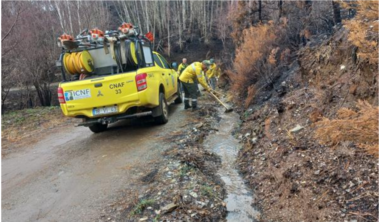
Figure 84. The Lama Grande fire covered more than 2 300 hectares of forest areas in Portugal and Spain on January 28 and 29, affecting the Montezinho Natural Park in the far north of Portugal. The prompt intervention of "storm patrol" teams before and during heavy precipitation days made it possible to protect the road network and substantially reduce the risk of erosion.
